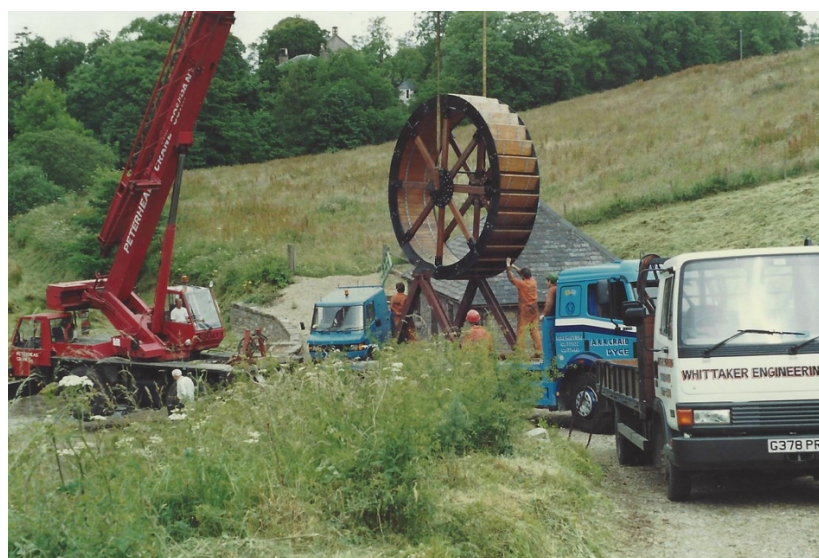
Photo courtesy of Ken Whittaker of Whittaker Engineering, Stonehaven, showing the new waterwheel Arriving for the Mill of Benholm during the extensive restoration works in the 1990s
