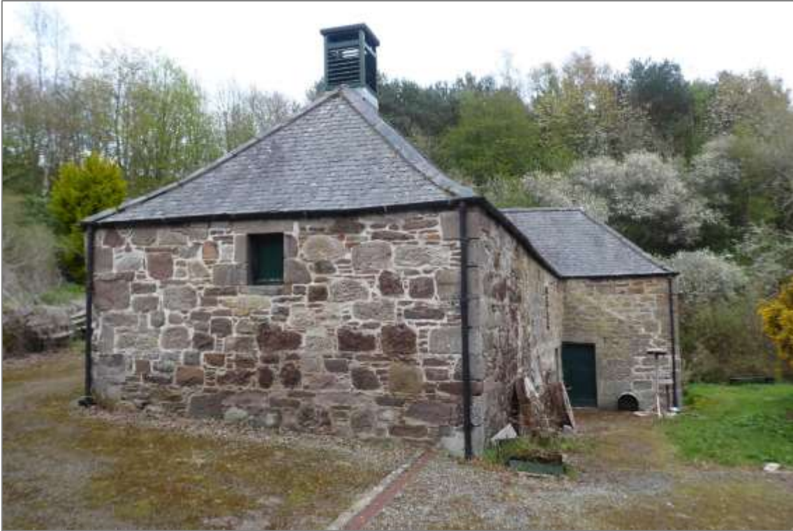
Mill of Benholm, meal mill west elevation showing the rebuilt kiln wall and opening into the drying kiln. Compare to Hume (1974) image at https://canmore.org.uk/collection/444642 .
