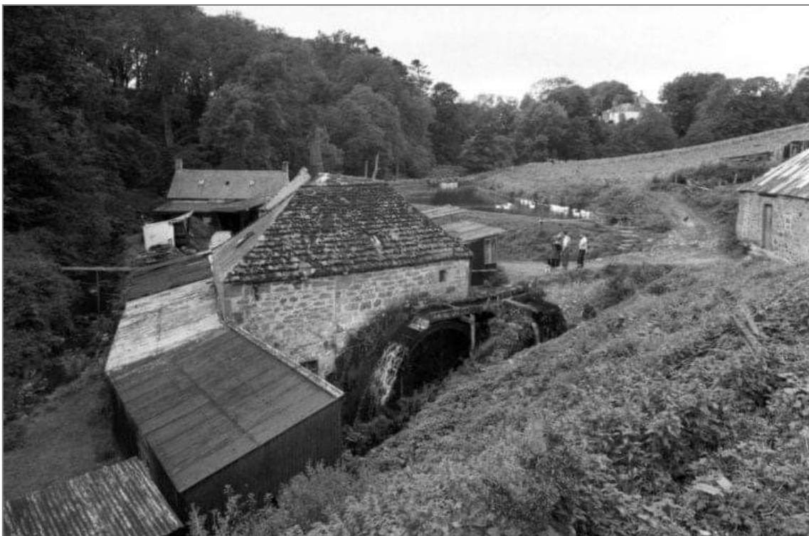
Mill of Benholm, photograph from 1970. Note the corrugated sheet roof over the grain store and no windows in the front elevation. Image by Ian Hardie in Aberdeen Press & Journal, 10 th Oct. 1970, courtesy of MoBE.
