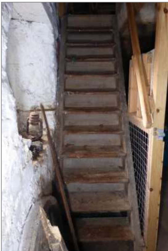
Mill of Benholm, timber stair with reused timber boards finished in earlier wallpaper.
