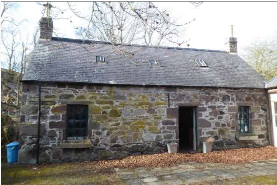
Mill of Benholm, miller's house front elevation in 2023. Note the symmetrical roof over the asymmetrical elevation. What may be the remains of a very small low window are located to the south of the current door.
