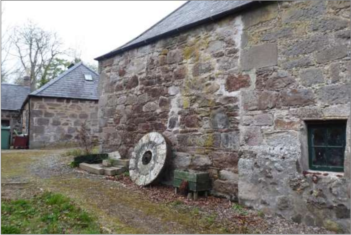
Mill of Benholm, meal mill south elevation showing the later kiln construction abutting the meal mill, note the large squared sandstone blocks and thinner levelling stones. Visible below the window is the older field stone rubble wall construction.
