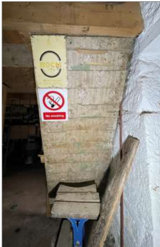
Mill of Benholm, timber stair with reused timber boards finished in earlier wallpaper.
