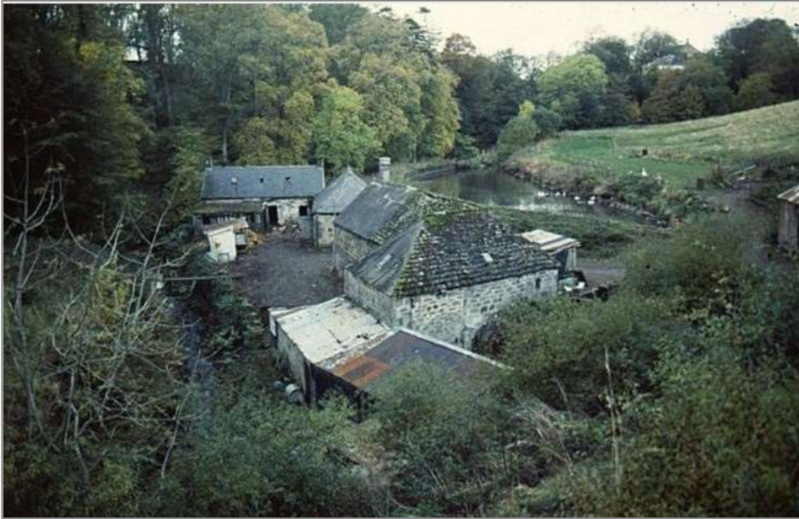
View of the Mill of Benholm in 1983 prior to adaptation showing its roof finishes including the earlier stone slates and later grey slate, note also the corrugated sheet roofs over the southern Engine House area. © Mills Archive Trust: JWN collection image 10742 https://catalogue.millsarchive.org/benholm
