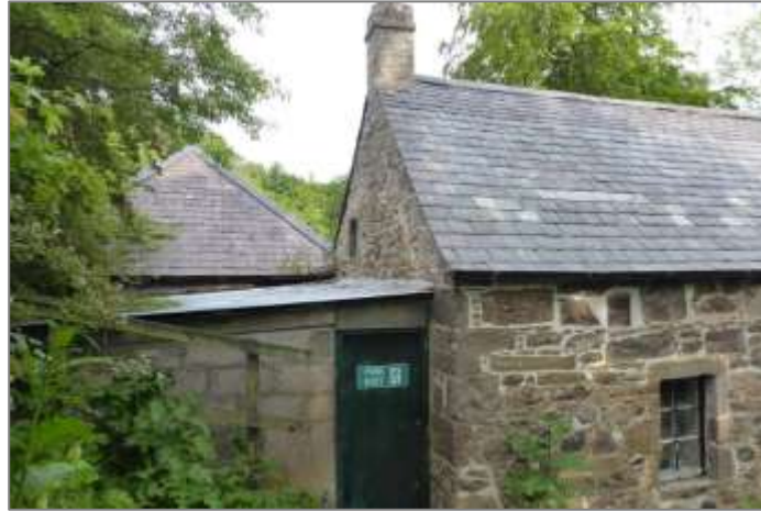
View of the kitchen extension abutting the miller's house and byre.
