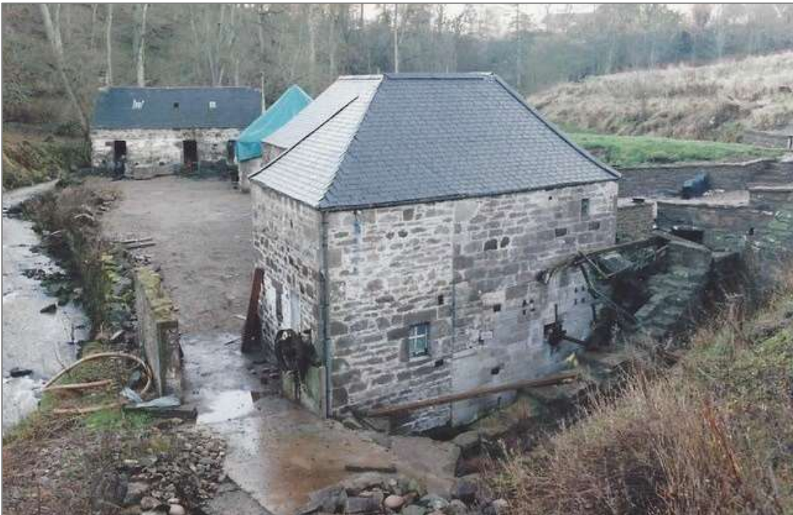
View of the east end of the meal mill (late 1990 or early 1991). Note the remnants of the waterwheel (wheel axle, wooden trowse), and on the left a freestanding stone wall, part of the southern extension, possibly dating to c.1900, now removed. The meal mill has been re-roofed in a uniform Welsh slate (WE Ltd files)
