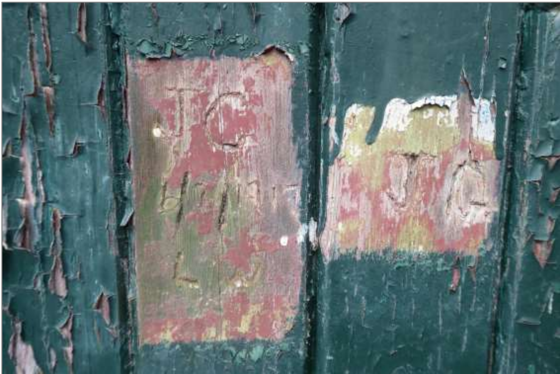
Mill of Benholm, meal mill south elevation, door graffiti dating to 1917.
