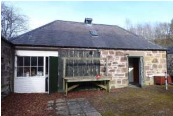
General view of the south elevation facing the courtyard.
