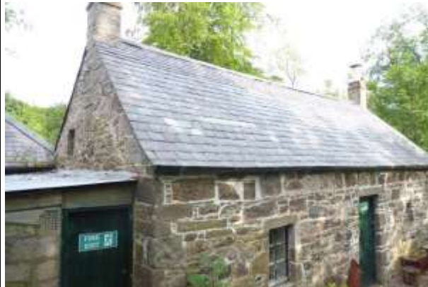
Probable raising of the wallhead seen on the rear elevation and also north facing gable where there is a protruding outline of an earlier lower and steeper gable slope.
