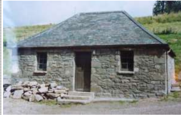
The grain store was one of the first buildings to be completed during the adaptation. It appears there was considerable reconstruction of the façade to introduce two windows and a central door. (HES file image, c.1992)
