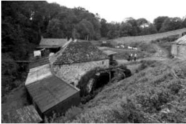
Mill of Benholm in 1970. Note the corrugated sheet roof over the grain store and no windows in the front elevation. Image ©Aberdeen Press & Journal, courtesy of MoBE.
