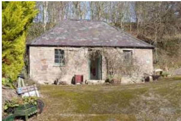
General view of the front (south) elevation.
