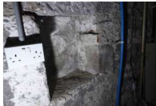
Two recessed openings on either side of the byre door may have been former openings but don't appear in the stonework externally.
