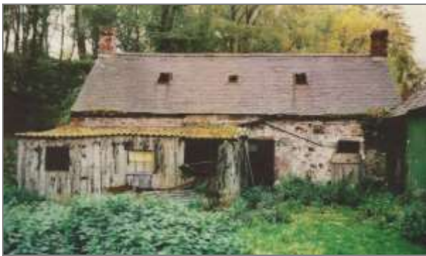
The miller's house in around 1986 note the timber and corrugated sheet extension probably added sometime from 1901 - 1923 (W&D DC postcard, © Aberdeenshire Council).
