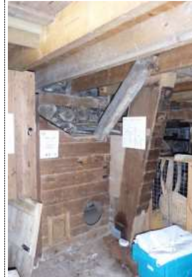
View of the Large Fanner . Groats are transported to the upper floor for grinding by the Bucket Elevator ; unshelled oats are blown into a second hopper with an outlet at floor level (bottom left).
