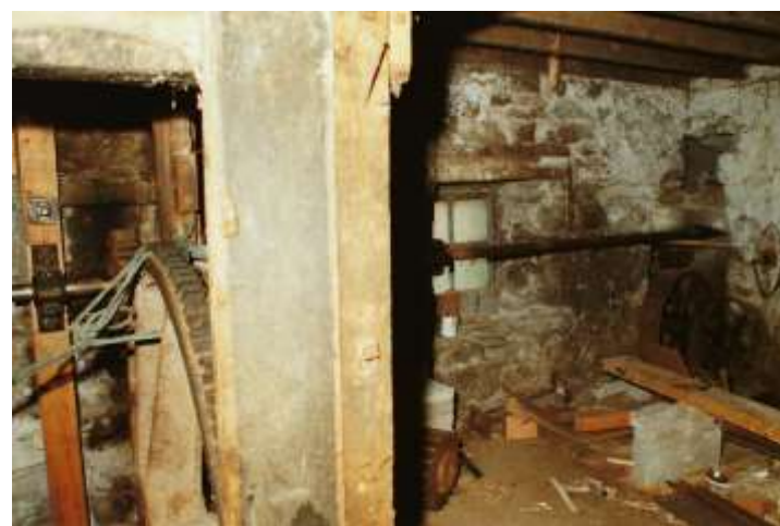
Similar view taken by WE Ltd during the restoration works. Note the Auxiliary Spur Wheel on the left, and its drive shaft behind already restored.
