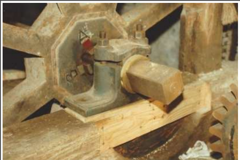
WE Ltd repaired hub on Auxiliary Spur Wheel (WE Ltd image).
