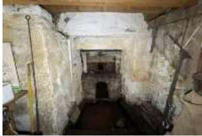
General view of the kiln fire box .
