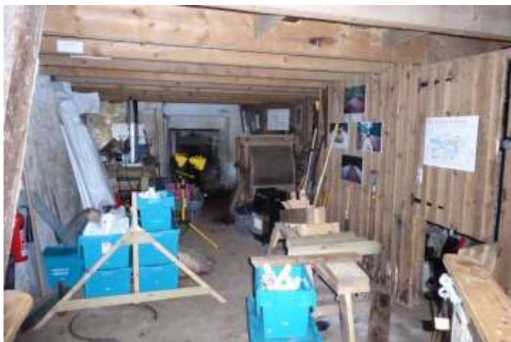
General view looking west toward kiln fire pit in 2023. The space is cluttered by storage of modern items not associated with the mill operations.
