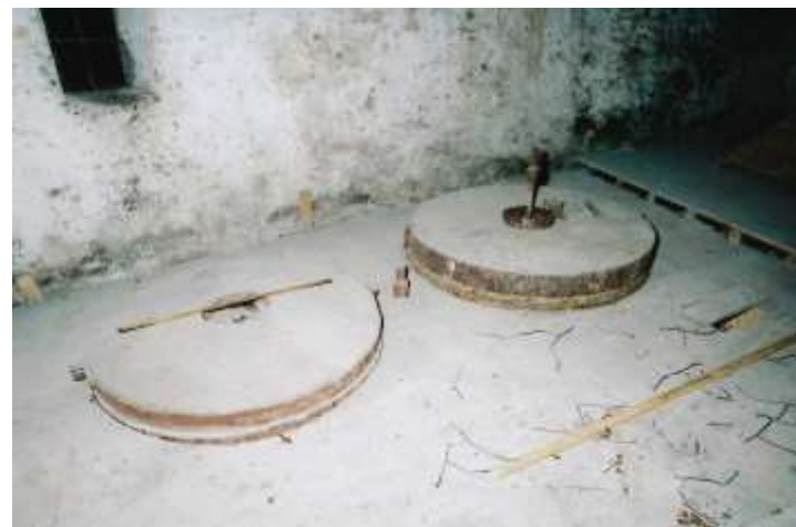
WE Ltd image during the restoration works, c.1991 with the milling stone equipment dismantled to allow repair and assessment of the stones left by the last miller.
