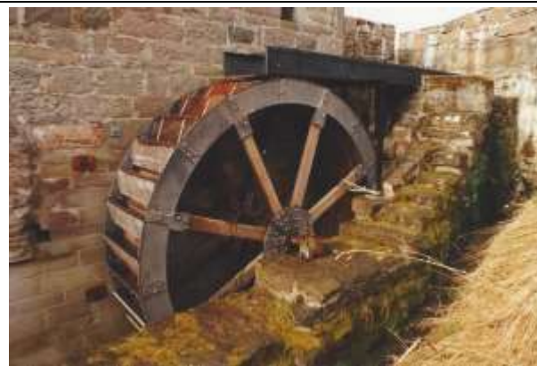
General view shortly after repair and renewal of the waterwheel, with the new Trowse clearly visible above the Waterwheel and a new higher boundary wall next to the building. (HES file image c.1992).
